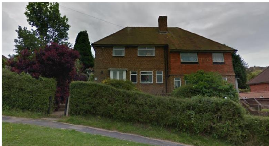
Fig. 5: view of Keymer Road from pavement level.
